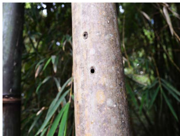
Figure 10: Holes in bamboo caused by insects (photo: Matthias Schöller)
